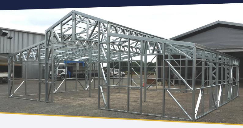
A classic design reimagined with modern technology, the CSF 110 Heritage Barn is a 110m2, pre-engineered, framed building, roll-formed from light-gauge New Zealand steel.
